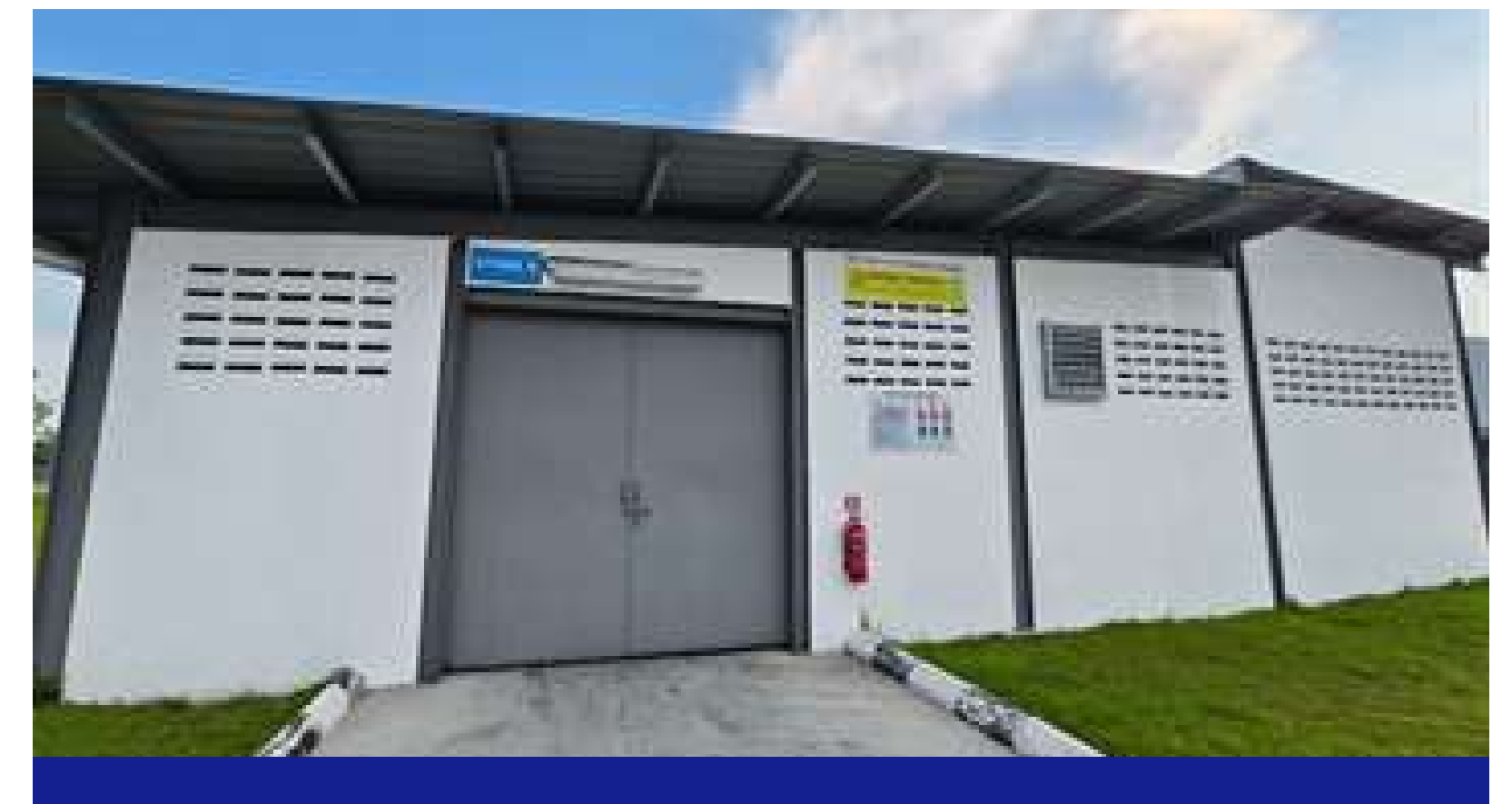
Scheduled waste storage in SunPower Malaysia
